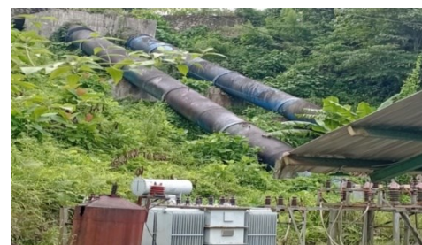
Gambar 4. Pipa Peast (Penstok)
